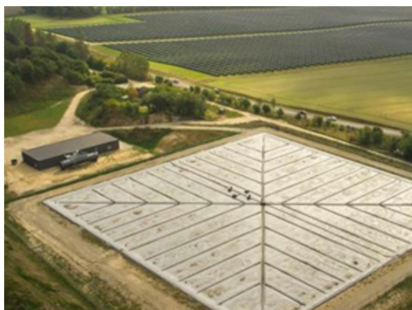
FIGUR 20: DAMVARMELAGER FOR SOLVARME I DRØNNINGLUND (62.000 M3)
